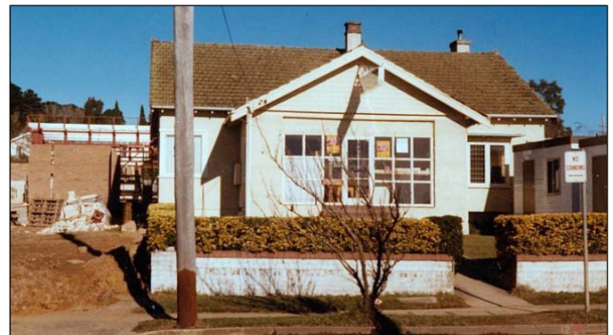
Office at 226 Argyle Street Moss Vale C1980
