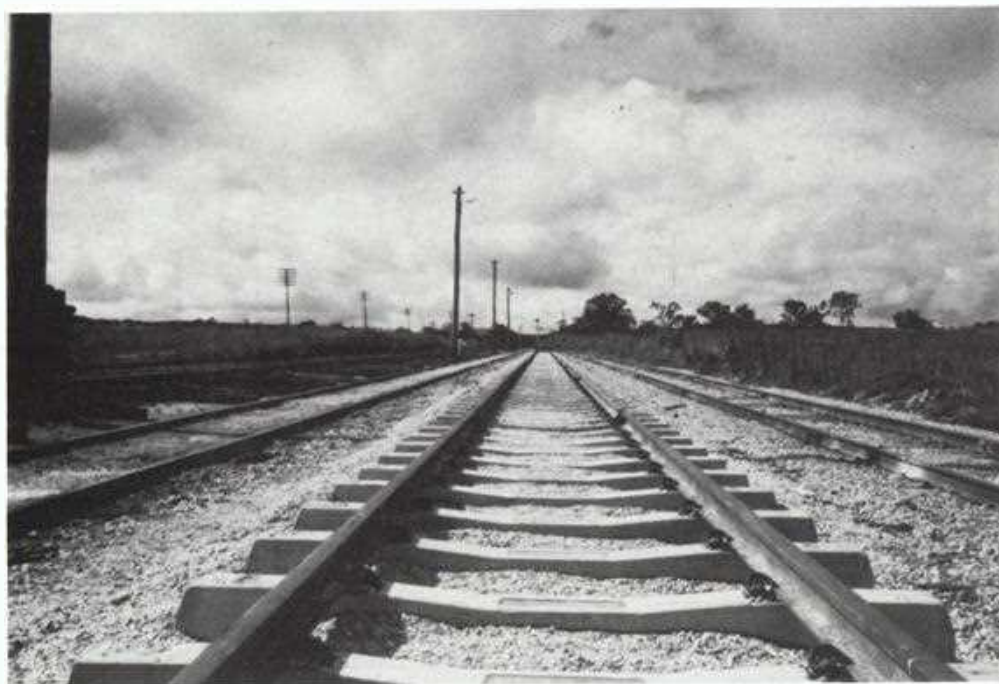
Concrete sleepers at Medway Junction
