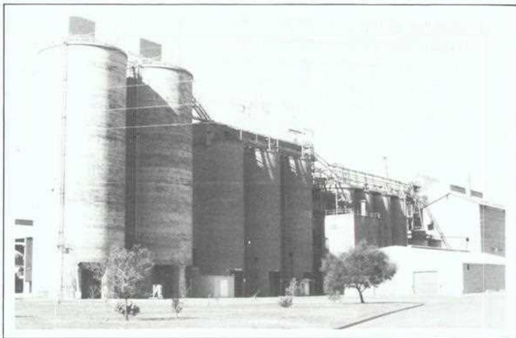
A grinding plant requires adequate storage for its product. Pictured are the five despatch silos with holding silos at the rear. On the right is the stock-house where the busy "bag trade" is carried out.
