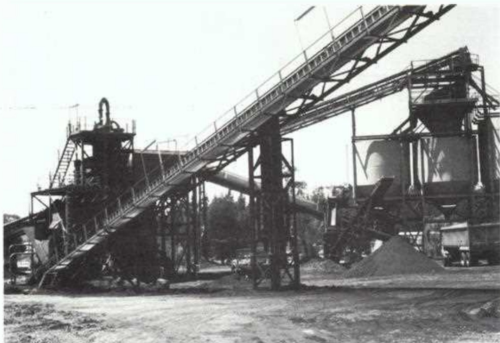
View of the washery (left of photo). Running across the centre of the photo is the coal conveyor carrying washed coal. The existing road bins can be seen in the right background.
