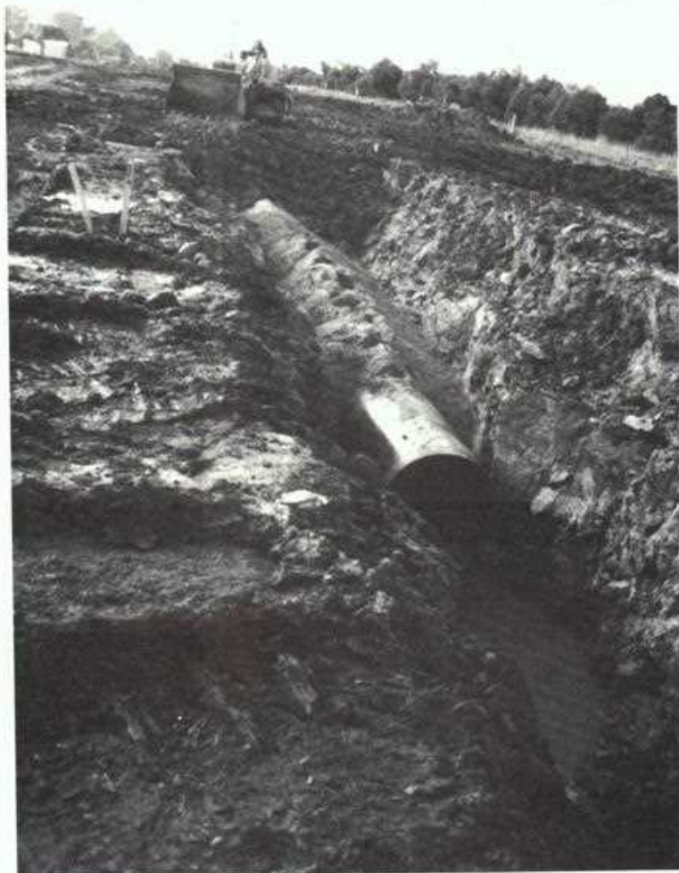
Backfilling over the new pipeline.
