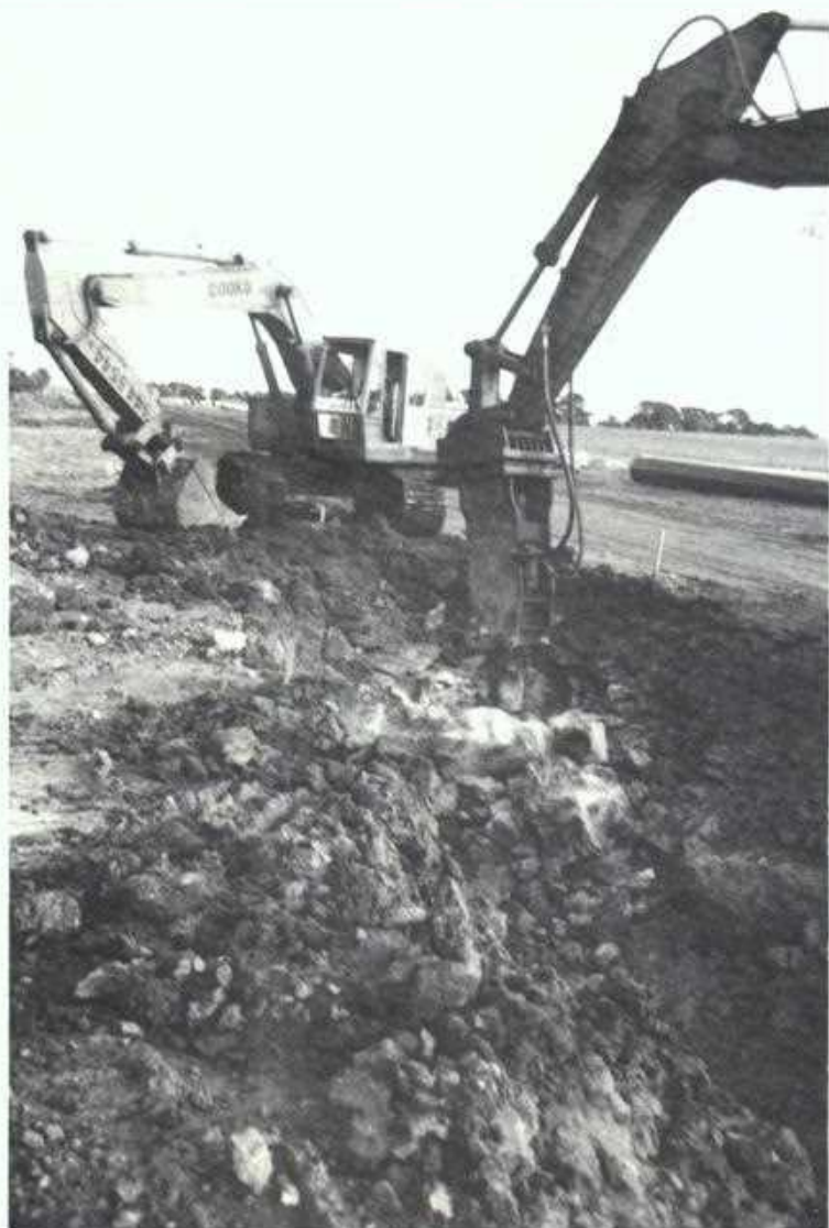
Hydraulic hammer breaking rock for the bed of the new pipeline.
