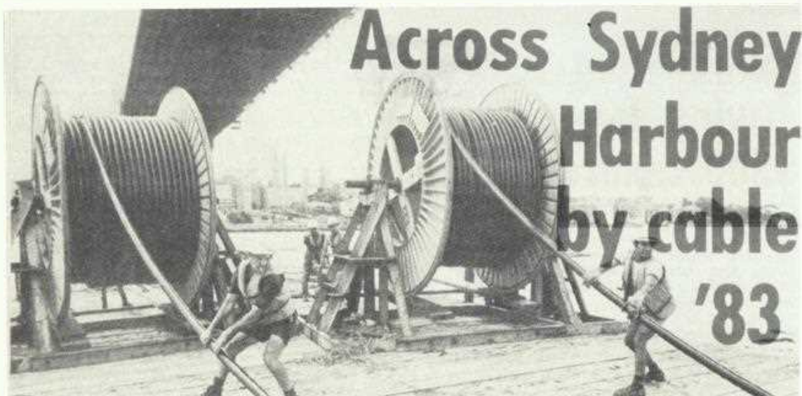
The cable being fed out during the laying under the Sydney Harbour Bridge.
