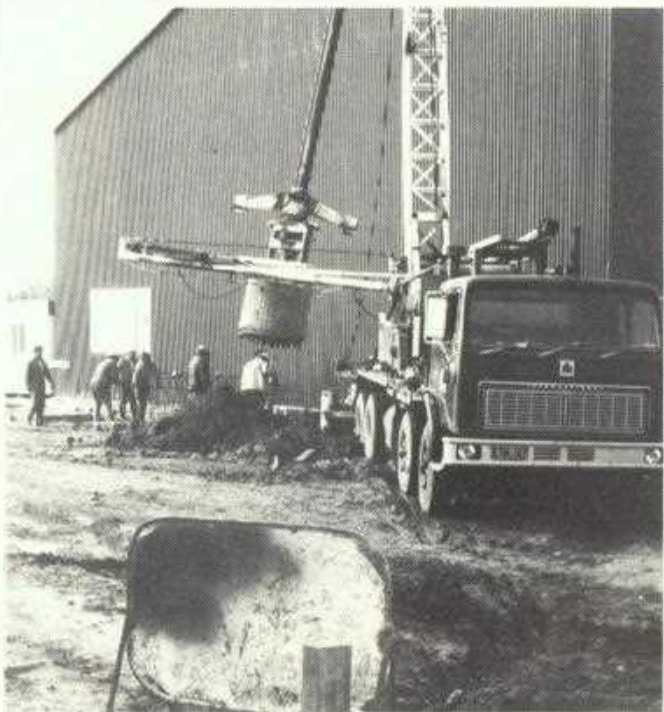
PREPARING for the piers for the fine grinding building ◆
