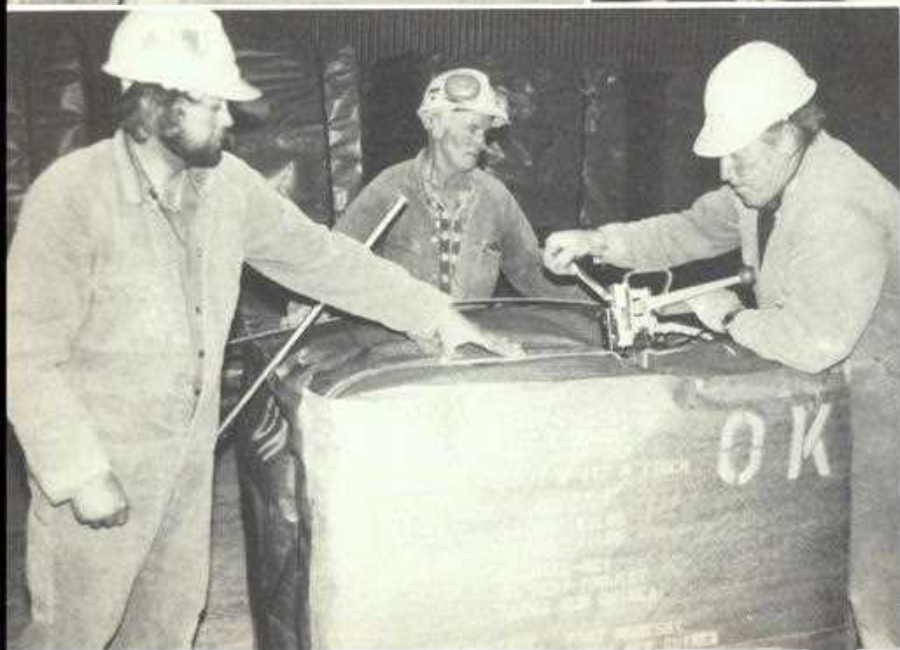
TOP LEFT: Jack Smith (left) and Ron McDonald taping the bottom plastic sheet to first layer of bags.
