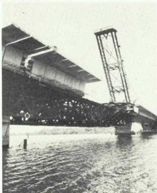
The erection tower and truss supported off the permanent structure (the pier in this photograph) eliminate much costly and unsightly false work during construction of the bridge.
