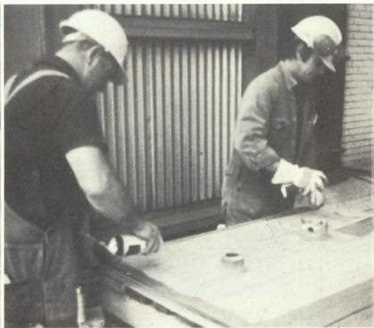
TOP LEFT: Jack Smith (left) and Ron McDonald taping the bottom plastic sheet to first layer of bags.
