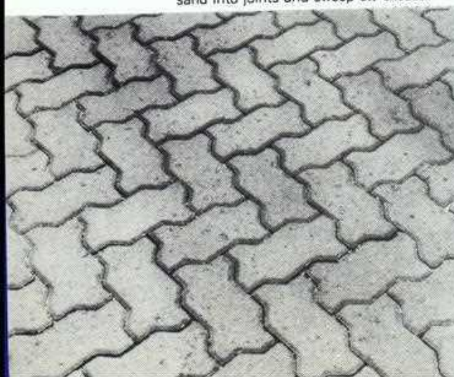
STEP 3: Spread fine dry sand over bricks, brush sand into joints and sweep off excess.
