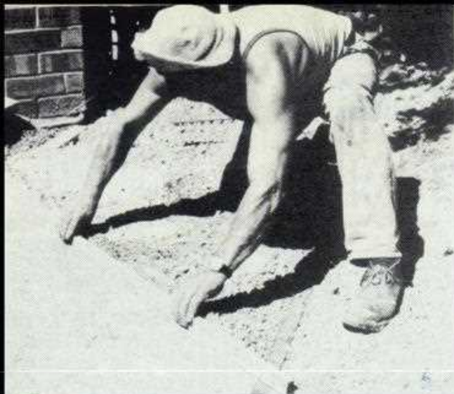
STEP 1: Prepare consolidated base. Cover area to be paved with 50mm sand. Screed sand to level required.
