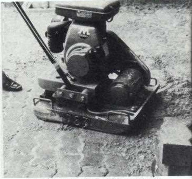
STEP 4: Compact bricks with hand tamper or preferably with vibrating plate until desired profile is achieved.
