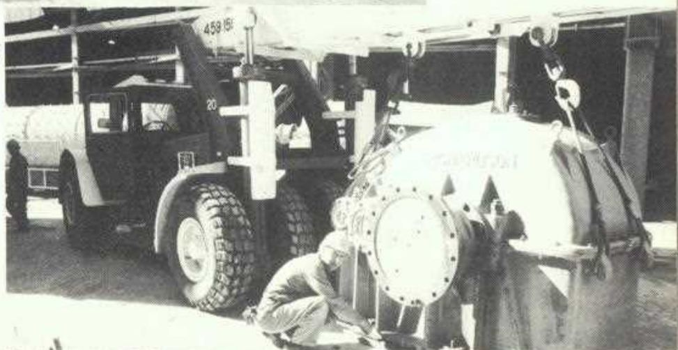
RIGGER John Rasins handling a slag mill gearbox. John's comment: "A piece of cake".
