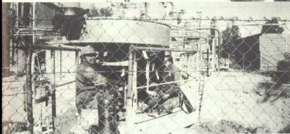
♦ MAINTENANCE — No. 1 sun and planet. While the hard slurry build-up is removed by bobcat, Gordon MacDonald and apprentice fitter Robert Wilson work on the gears.
