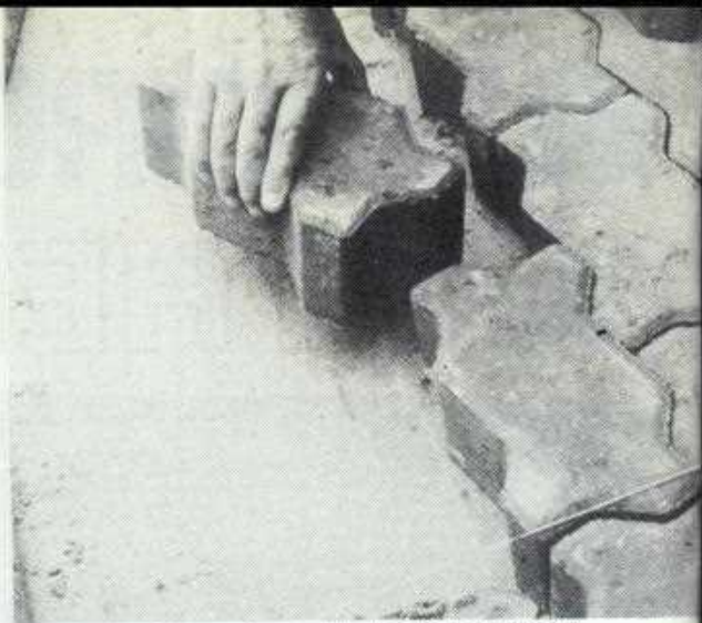
STEP 2: Select pattern and lay bricks to pattern on sand base, butted as closely together as possible.
