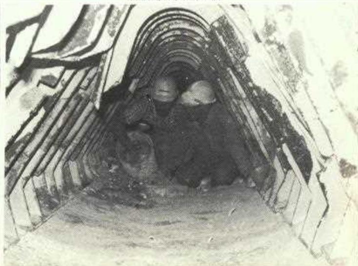
• TOM Marshall and Col Glacken repairing refractories.
