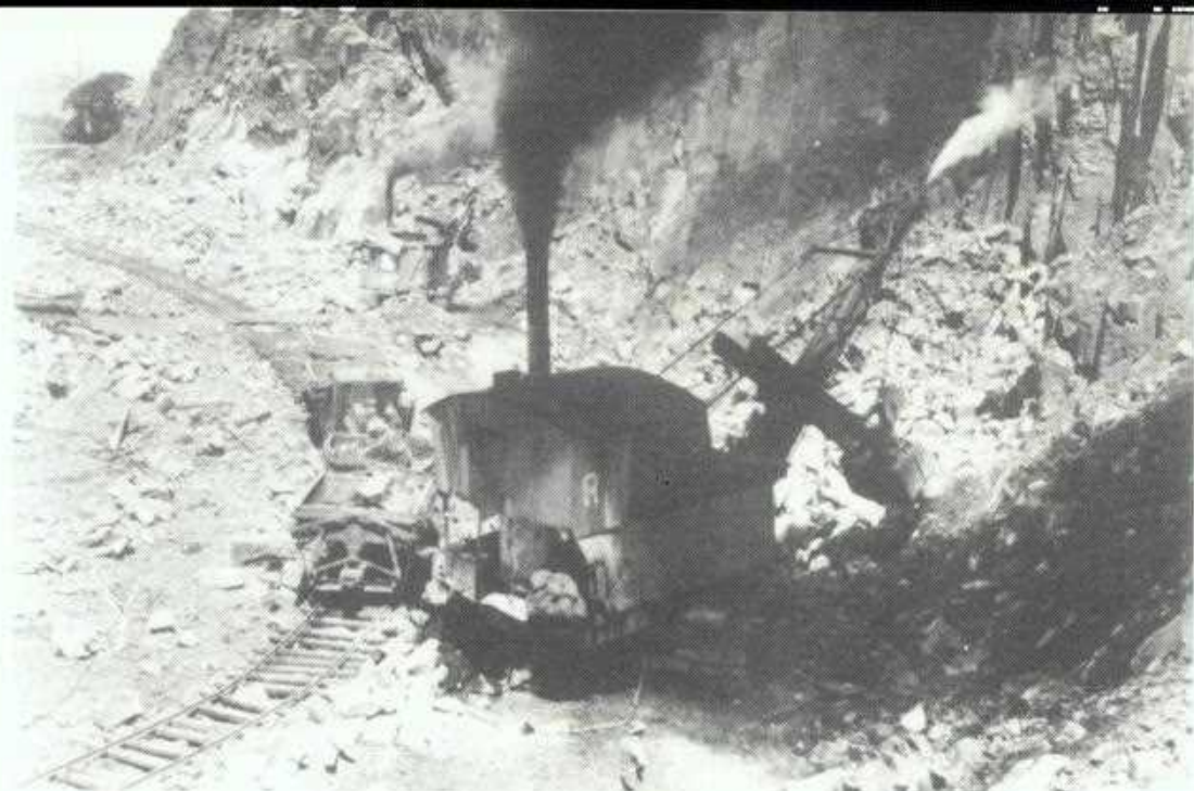
THE standard gauge blue metal quarry railway and on it can be glimpsed 'Wonga', an 0.6-OST Barclay product. The rough nature of the line at this point was normal as this section (near the face) was portable.
