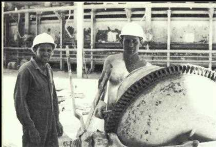
• BILLY Lamb and John Paull mixing the refractory.
