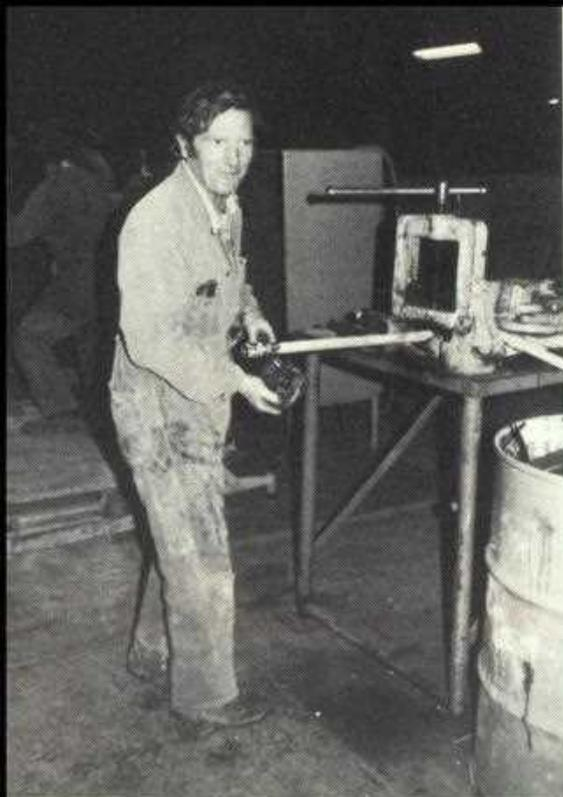
◆ FITTER Bill Toohey threading the end of a pipe in the Mechanical Workshop.
