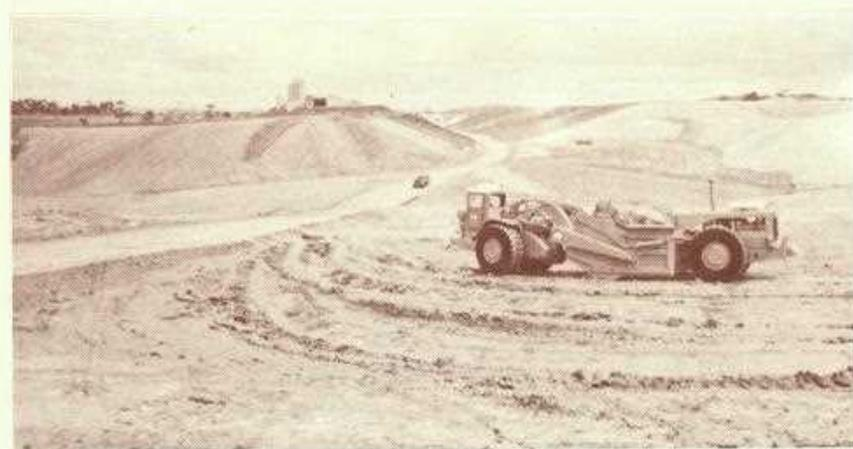
*TEREX scraper at work in the quarry. In the back-ground the overburden has been replaced and seeded.*
