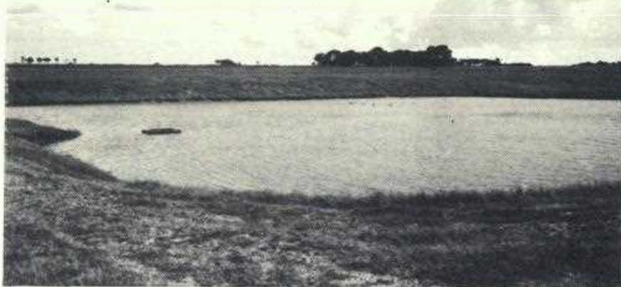
*Settling ponds east of the Works collect quarry silt.*
