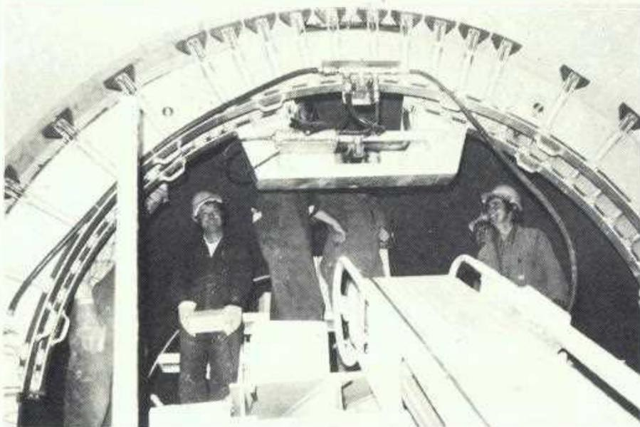
*DURING February the kiln at Wearn Ponds was shut down for nine days to enable the replacement of approximately 16 metres of bricks. Above is a close-up picture of the Mult-o-Ring with a group of production employees working as a team to get the job done.*
