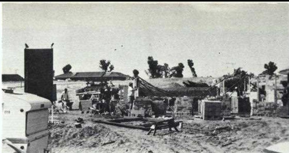
◆ **FIRST DAY:** Concrete foundations were laid and a start made on brickwork.
