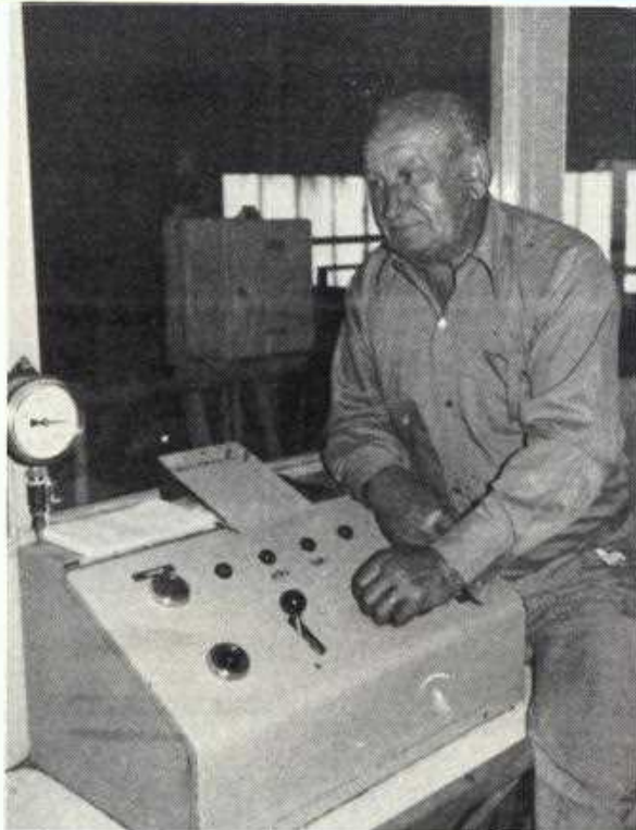
Crusher attendant Jack Parry with over five years' service concentrates as he operates the controls of the bridge gates over the hopper that receives the stone from Terex units.
