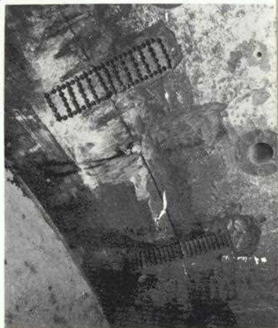
The picture above was taken inside the No. 1 cement mill and the picture below shows the same position on the outer side of the end plate showing the masterlock process in progress.
