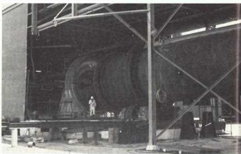
Top left: The two new sections for the kiln. Above: The firing end of kiln to be replaced. The picture shows the tracks set for removal of the section and support legs under the remaining section. Below left: The new section of the kiln ready to fit into place at No. 2 tyre station. Below: A close up of new firing end section.
