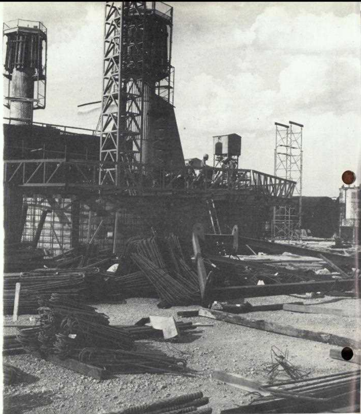
Start of construction of the four-stage cyclone pre-heater tower at Berrima.
