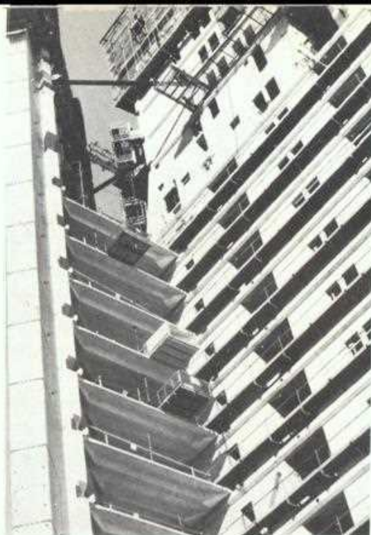
This end elevation photo of a main column shows support of column to service core by part of prestressed flooring system.
