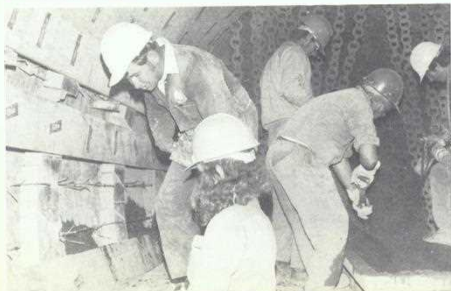
● Blocks covering chain spiral and steel sprigs used to bond material.
