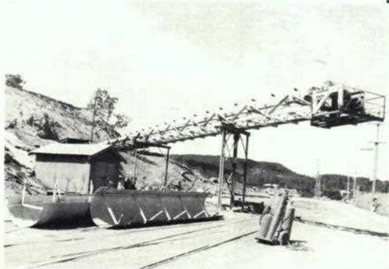
Nearing completion at Charbon works is our coal conveyor, which we hope soon to show you in action loading rail trucks.
