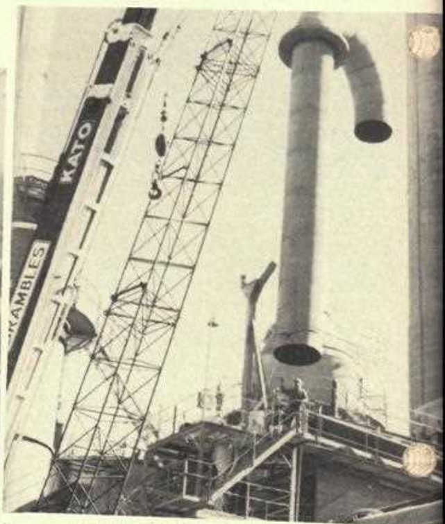
BELOW: Erecting No. 1 kiln flue ducting.
