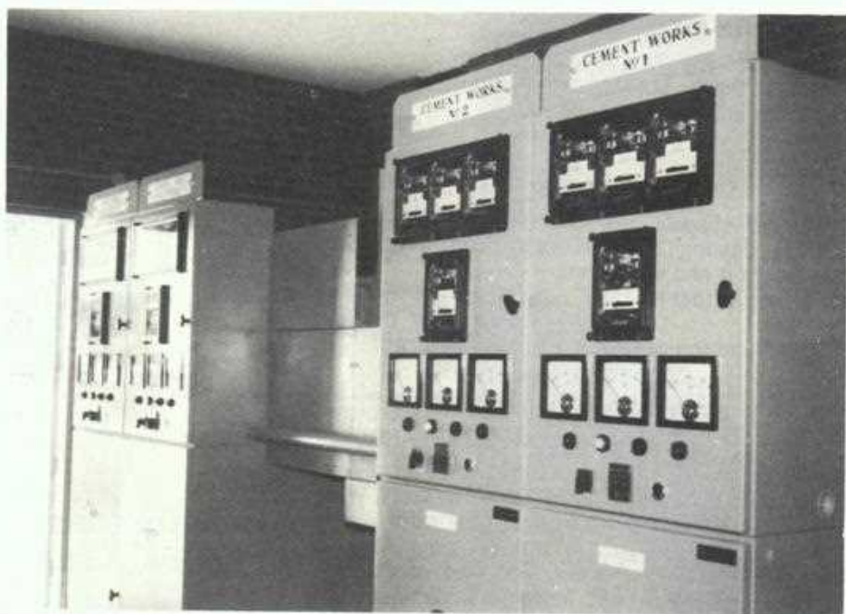
Along with the upgrading of the plant machinery, our Electrical Department were pleased to see the installation of a new incoming sub-station (above) and the replacement of the high voltage switchgear at the cement mill sub-station. (Below) Bill Purdy, Works' Carpenter, uncrating the switchgear before installation.
