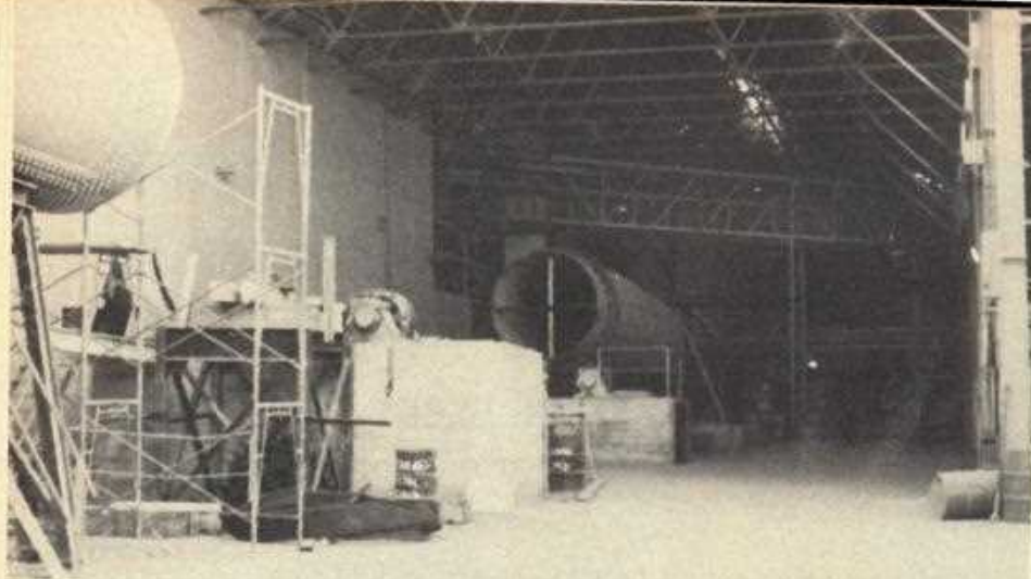
BELOW: Erecting No. 1 kiln flue ducting.
