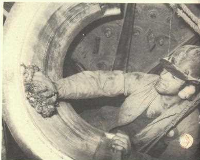
BELOW: Fitter Trevor Hodgson preparing Raw Mill bearing for blueing.
