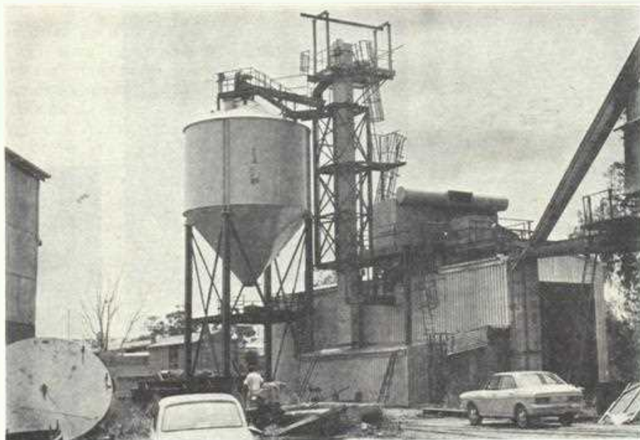
This bulk handling facility is being erected in the Brisbane suburb of Rocklea. It will be used for unloading and storage of lime for distribution in Brisbane. The plant includes a rail frock hopper, screw conveyors and bucket elevators. It is also equipped with a large dust collector to ensure dust free operation. Installation is almost complete and it will be in operation in January.
