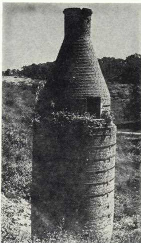
This old vertical lime burning kiln at Portland used to be hand fired with wood.
