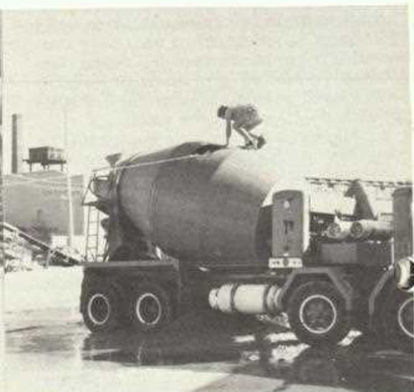
2. Cement plants and distribution depots have their problems, but so do the customers. Pictured is a premix Agitator fully loaded with 8 cu. metres of concrete and a broken gear box on the discharge motor, preventing unloading. A race against time (setting time) is involved. To get the concrete out of the mixer, a hatch plate has been removed from the Agitator drum, and a rope attached to a tractor to turn the hatch to the bottom. The concrete is then hosed out and dumped as a total loss.
