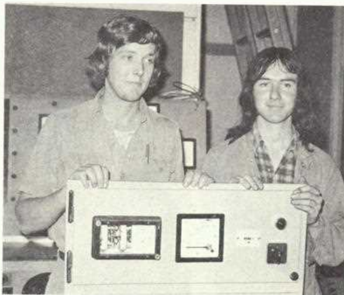
Above: Electrical fitter Bernie Rowley and his Apprentice John Bath with some of their handiwork. Made from one-sixteenth inch steel plate, it is a new panel fascia for a new service pump in the Power House.
