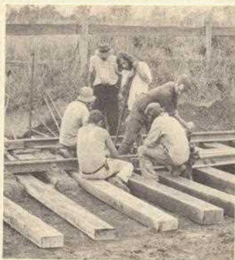
Above: — Putting fish plates on the new crossing.
