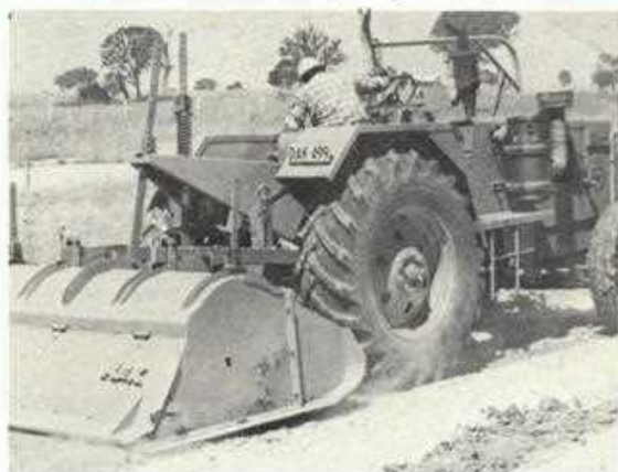
A Pulvimixer mixes the lime into a road base material.
