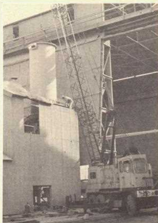
Above:— Careful manoeuvring was required to place the shell in its final position.
