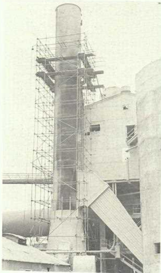
The stack with the scaffolding partly erected.
