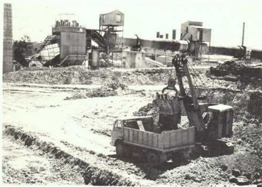
Loading Clay Shale at Berrima No. 5 Precipitator and Kiln in the background.
