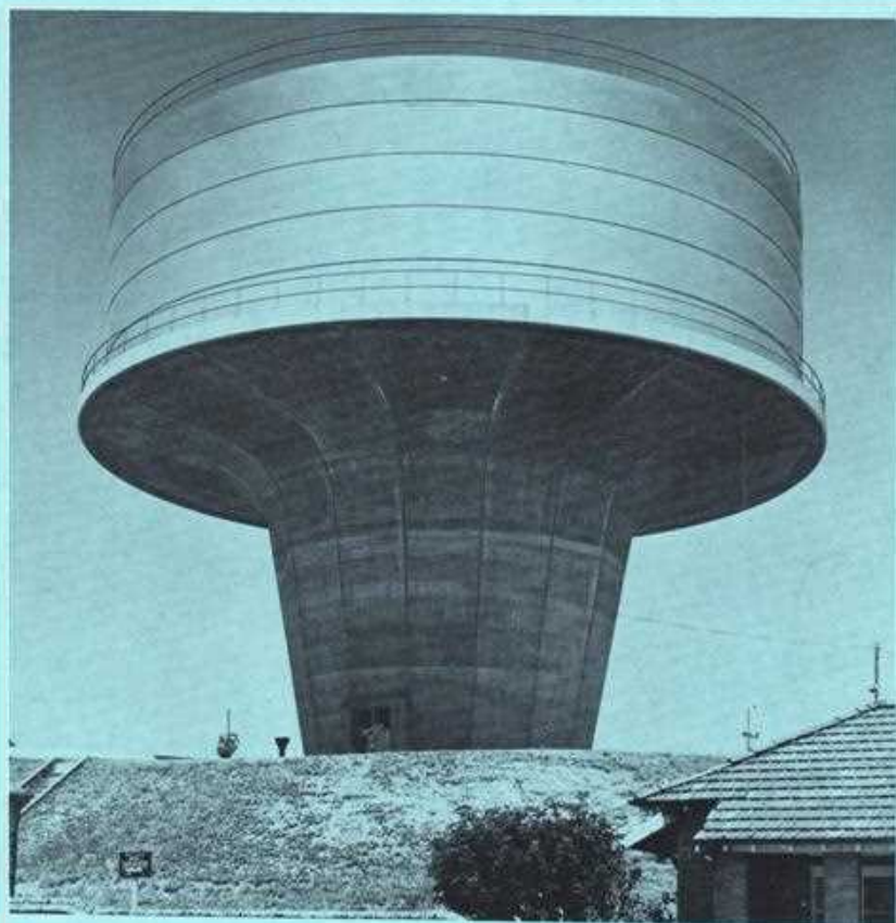
Petersham Elevated Reservoir — More Southern Cement. It consists of a concrete base with a one million gallon steel tank on top. The concrete pedestal is fifty feet high and just over ninety feet in diameter. The concrete was Ready Mixed.
