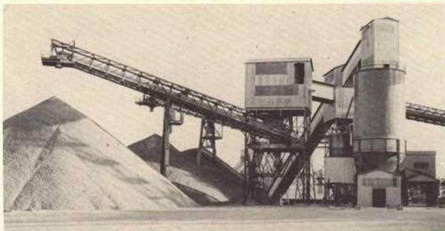
Marulan — Part of the hydration plant and stockpiles.
