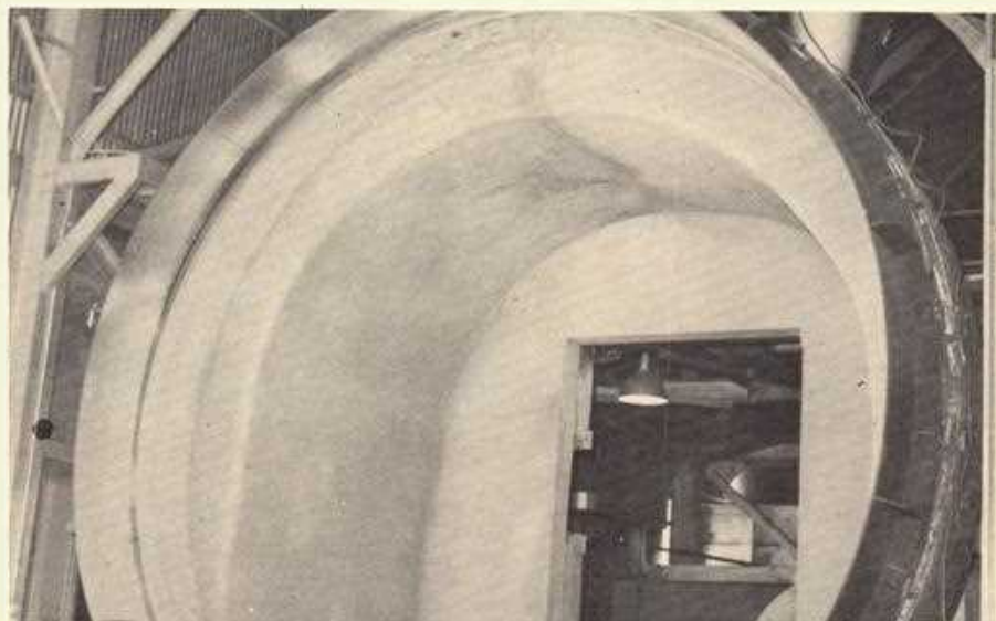
The kiln head was relined, but instead of the usual refractory brickwork, a castable material was used. This should result in improved wear resistance at lower cost.
