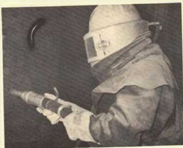
A contractor wearing special protective clothing, prepares to "Sand" blast No. 1 Cement Mill Shell.
