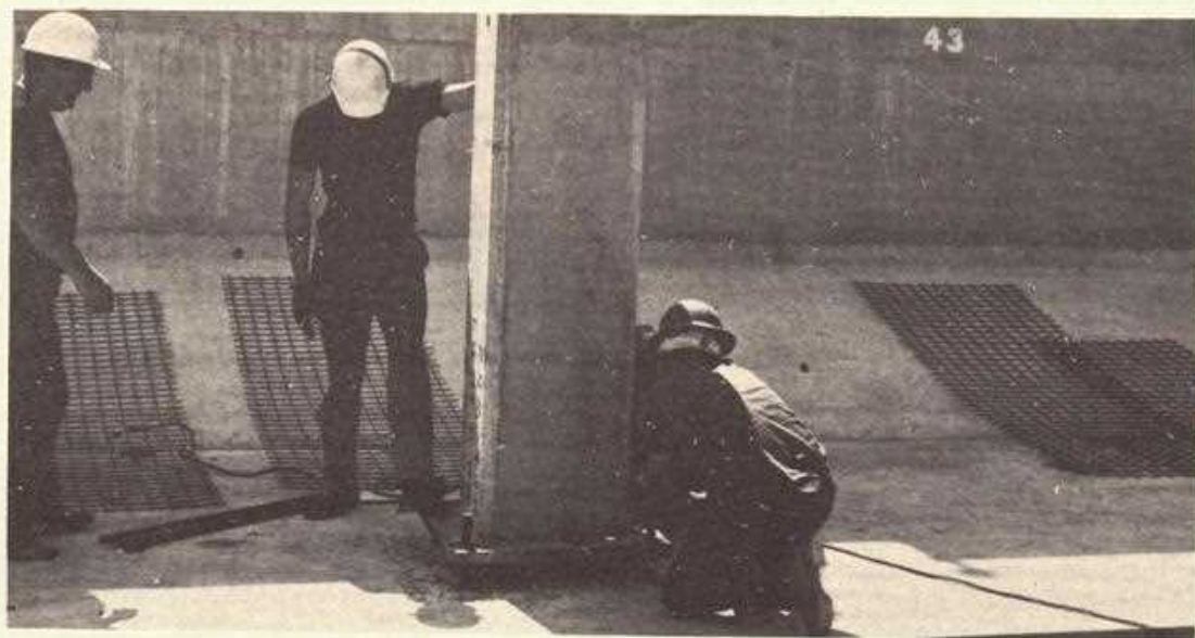
This shows work being carried out on the Maroubra Reservoir, which is 580 feet by 386 feet, with a capacity of 30 million gallons. A site plant was used for the 50,000 cubic yards of concrete required, and again Low Heat Cement was used.
