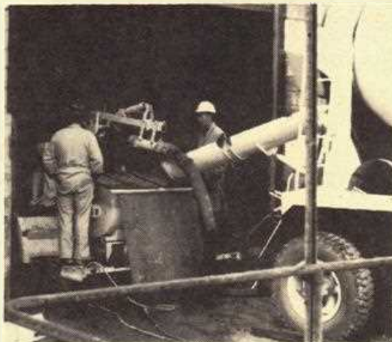
Concrete mixer feeding the pump during the pouring of the foundation of the 7.5 meg. Turbo-alternator at the Power House.
