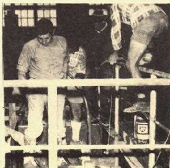
Concrete mixer feeding the pump during the pouring of the foundation of the 7.5 meg. Turbo-alternator at the Power House.
