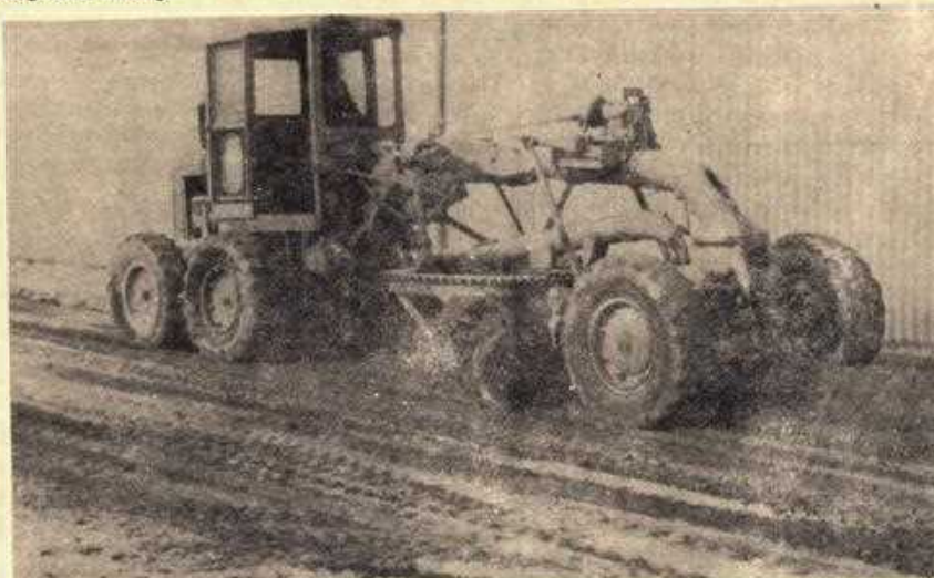
Lime spreading and mixing
