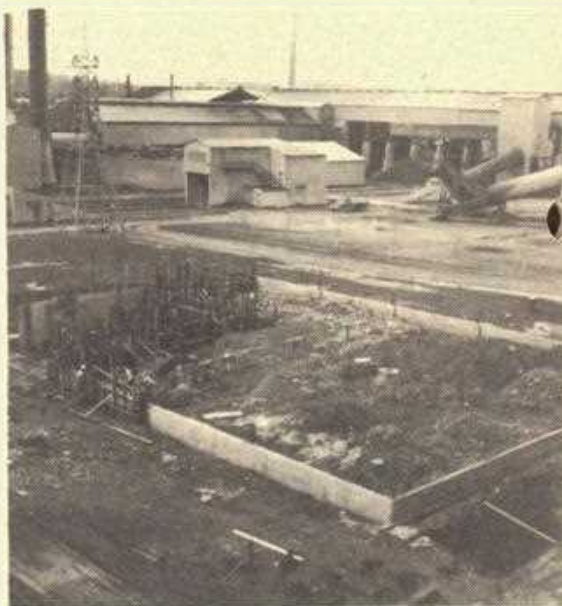
Foundation work on the new Laboratory. The basement storerooms and foundations are now completed, and the floor is being prepared.
