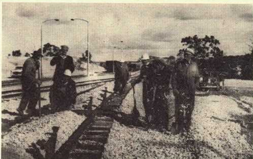
Marulan fettlers carrying out maintenance on a section of the line below the bins. Kneeling on the left is Albert Quail and on the right Jack Marsh.
