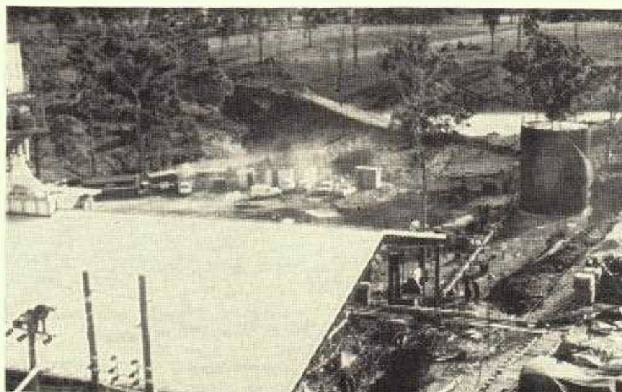
A section of the almost-completed Lime Burning Plant showing the 125,000 gallon furnace oil storage tank with the water storage dam in the background.
