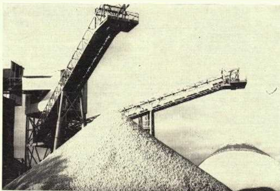
The stockpiles of limestone at the Calcimatic Lime Burning Kiln, showing the two conveyors which feed them.
