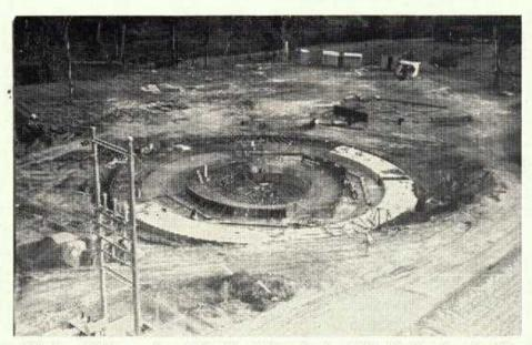
This is a bird's eye view of the foundations for the Calcinatic lime burning kiln at Marulan South. The photograph was taken from the top of the loading bins. The kiln is situated on the western side of the bins.
