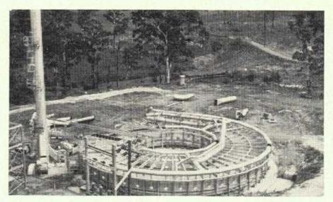
Construction of the Calcimatic Lime Burning Kiln and Hydration Plant at Marulan South is making good progress. The new earth dam can be seen on the right of the picture.
