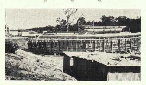
Good progress is being maintained on the Calcimatic lime burning kiln at the Marulan quarry. Erection of the steelwork is expected to start this month.
