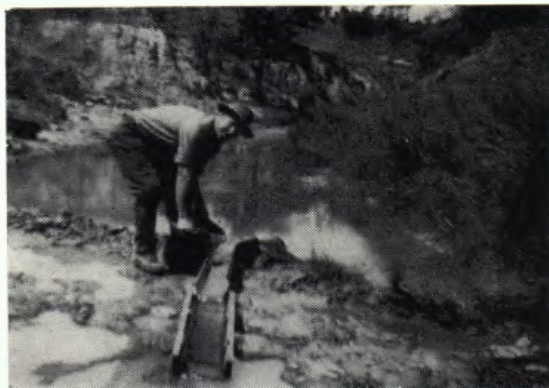
Gordon Bryant beside the sluice box with a pan of dirt ready to be washed.
