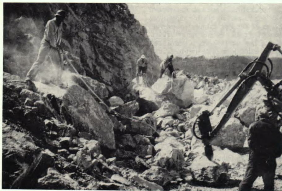
A new type of Jackhammer was demonstrated at the quarry. It was mounted on a tractor which also could be used as an end loader. In the background are regular Jackhammermen Hec, Johnston and Powderman Jack Watterson loading the pops.
