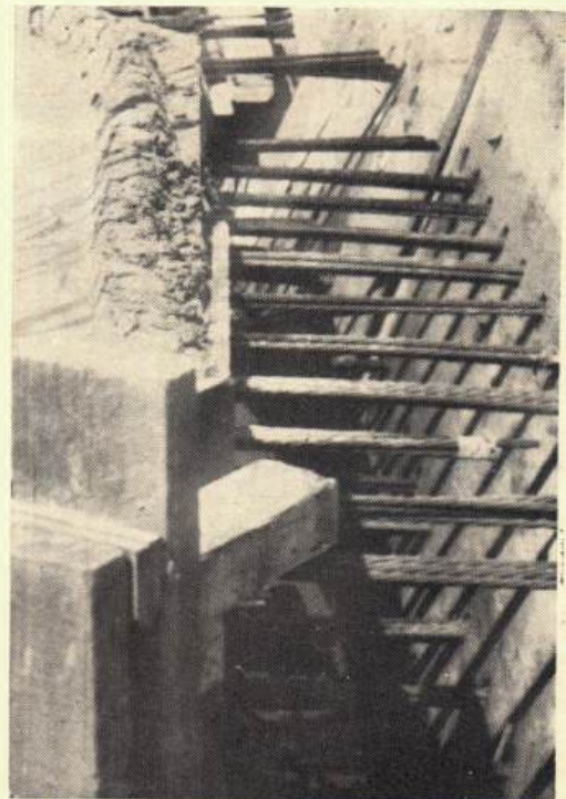
Cables protruding from slab.
