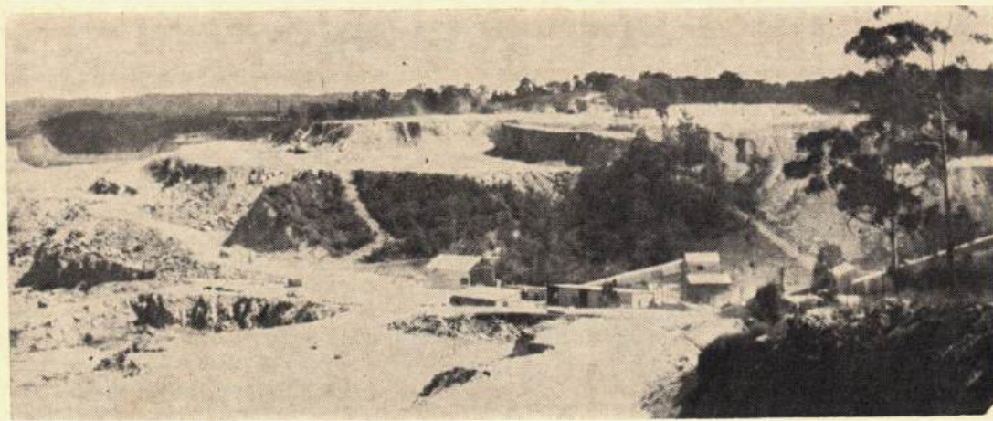
The Marion Shovel on the top bench in the background recently completed moving a hill. During the operation of about 6 months, it moved 1,129,770 tons. The rapid development and changing of quarry terrain can be judged from the photograph.
