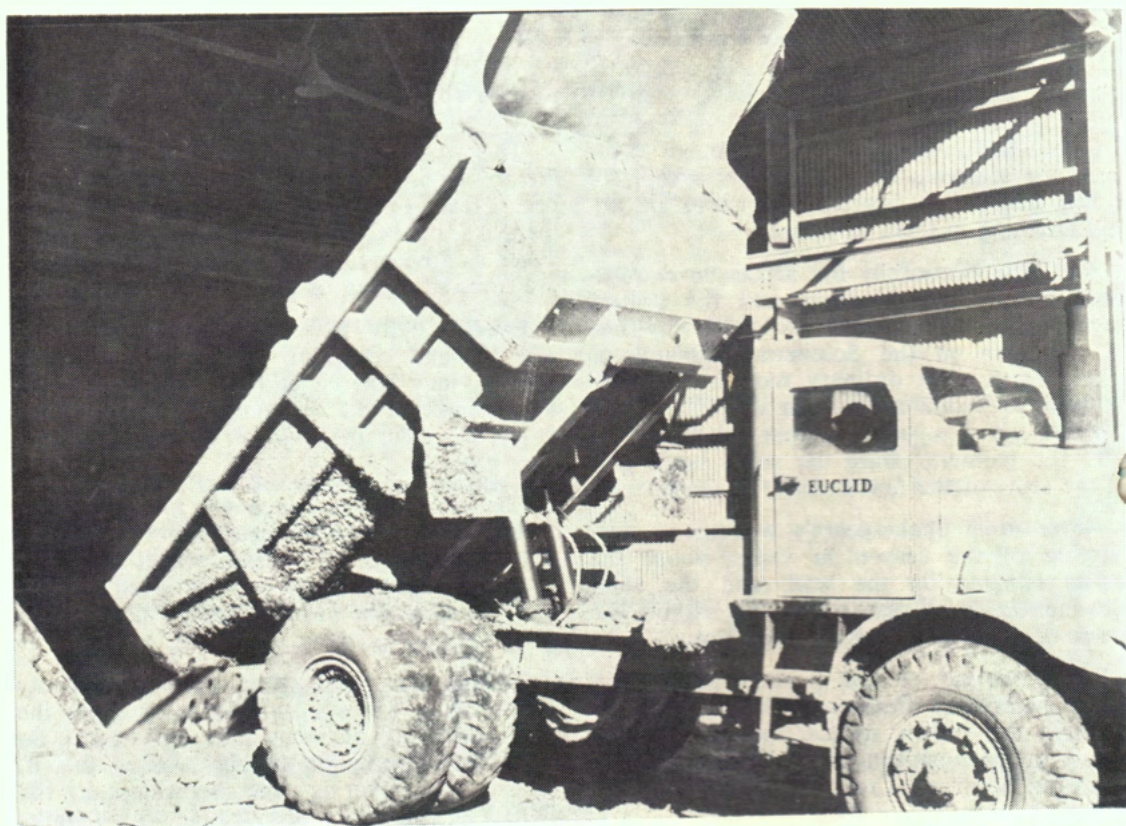
A Euclid dumps its load into the jaw crusher.
