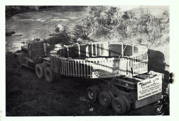
One of the major components of No. 5 kiln to be delivered last month, a kiln tyre. This is the first of 7 to be delivered and required special handling at Bargo River, being too wide to negotiate the Bridge.
