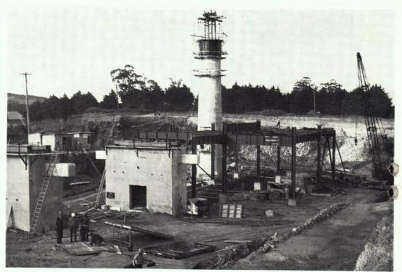
Steelwork commencing to rise from the foundations at discharge end of No. 5 Kiln with cooler stack in background.
