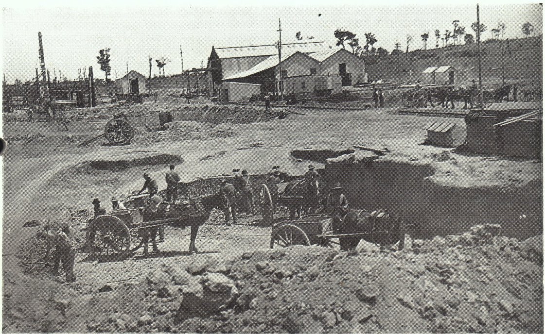
Now here's a gem! The excavation for the cement silos — by pick and shovel!!
