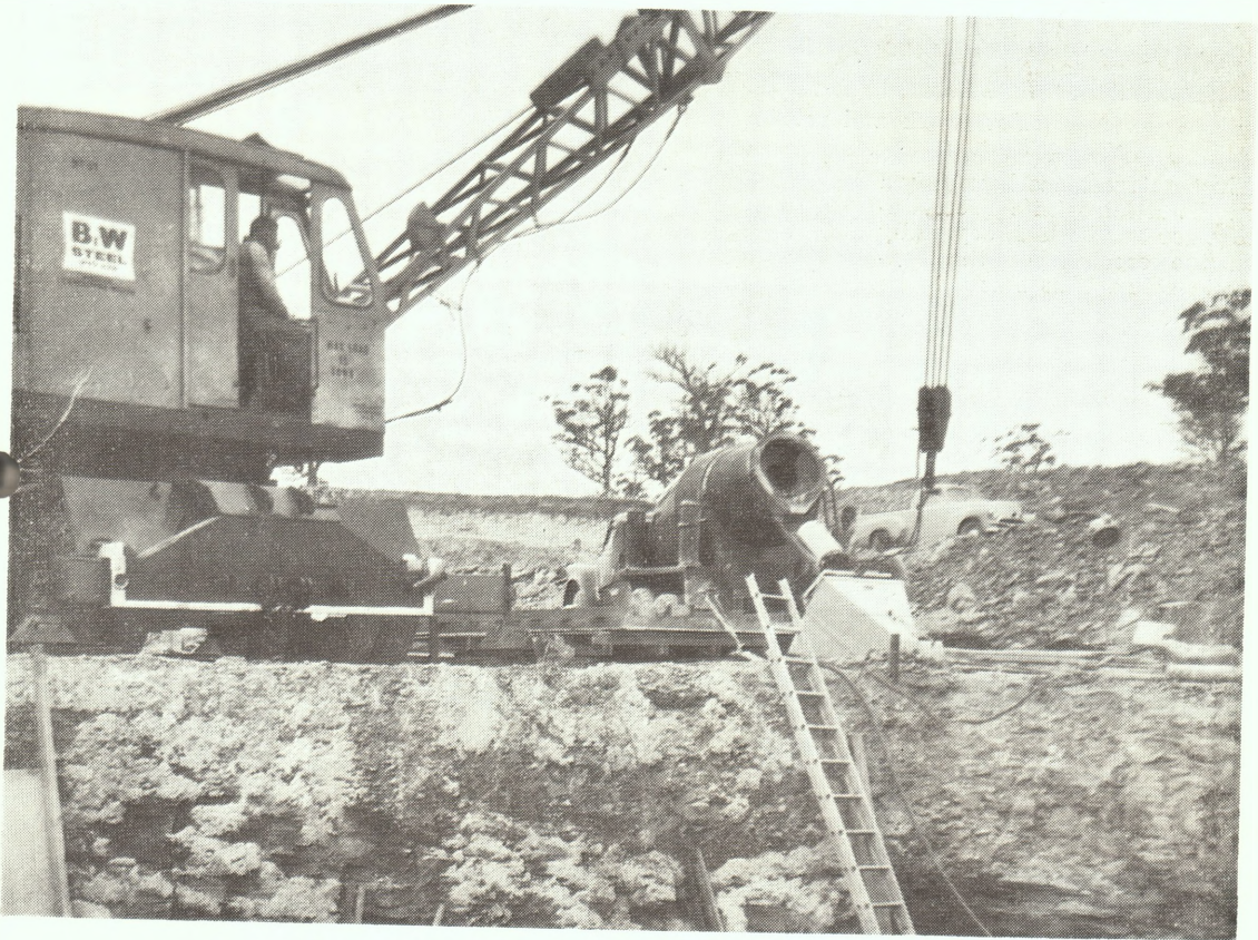
The above photograph shows a mobile crane at the edge of one of the No. 5 Kiln foundation excavations. With it is a ready mixed concrete mobile hopper.
