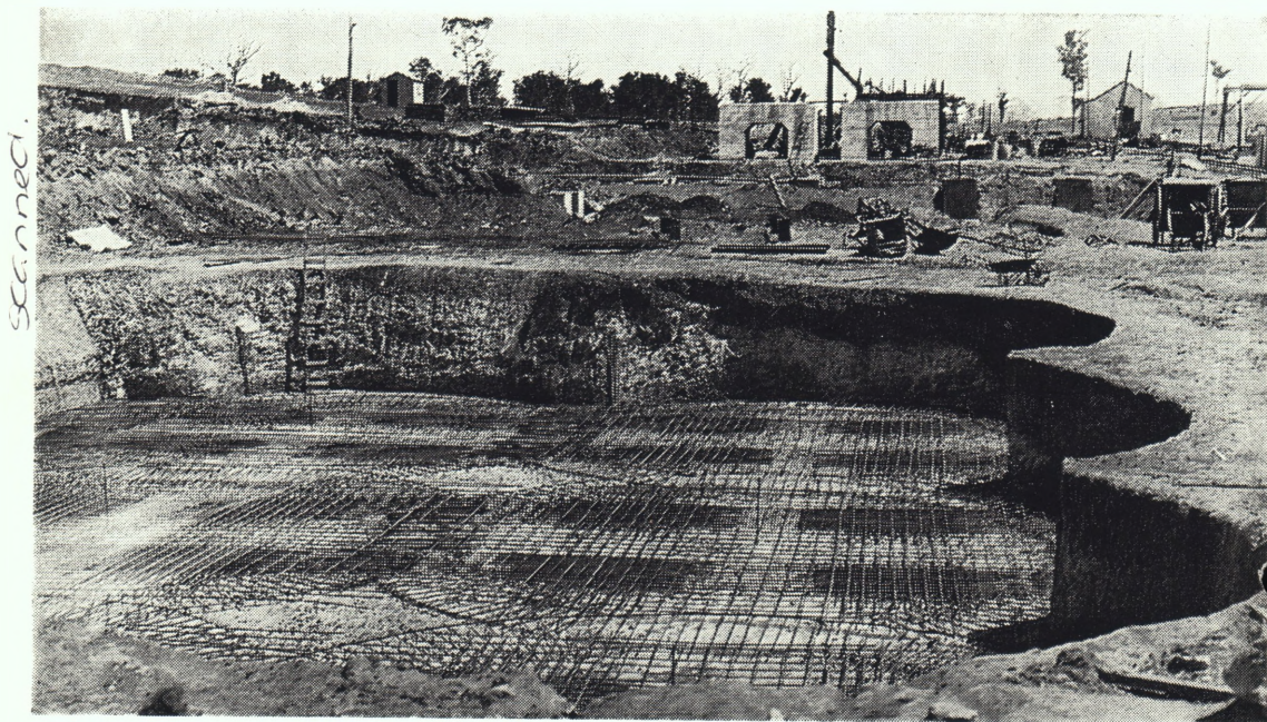
One month later! The pick and shovel boys have completed the silo excavations.
