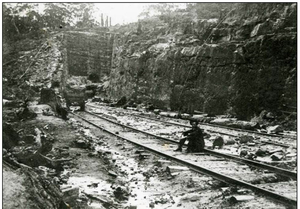
Tunnel construction near Yerrinbool for the Bargo deviation, c1915
