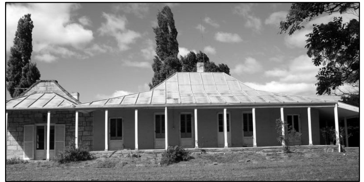
Wingello Park homestead, built 1840s
