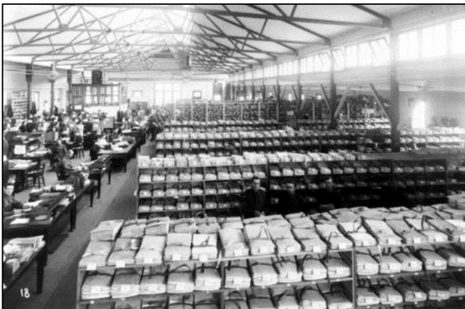
Files like sandbags at Base Records c1919 AWM DAX2211
