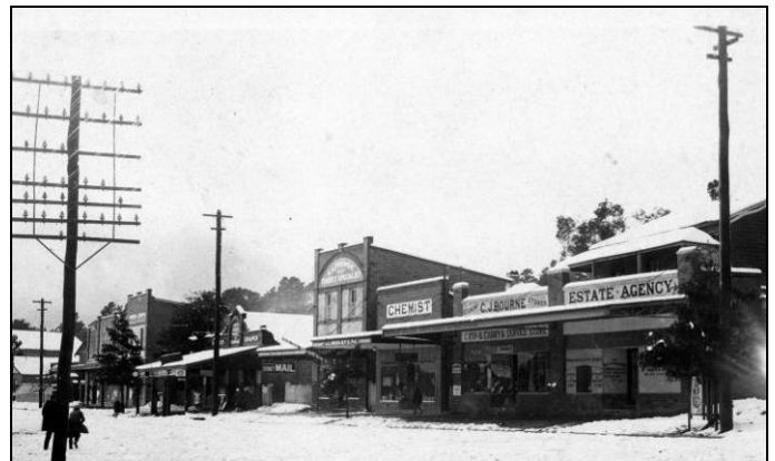
Railway Ave, Bundanoon after a snowfall showing telegraph (left) and electricity poles (right)
