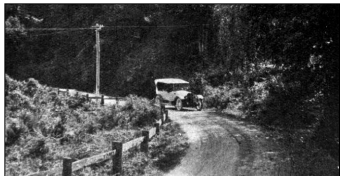
Electricity power pole on Barrengarry mountain road
