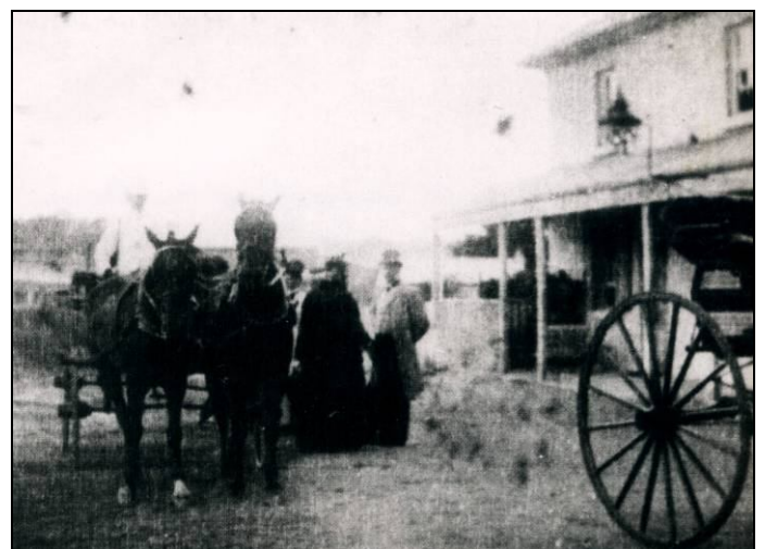
Travellers in Berrima at the Surveyor-General Inn.
